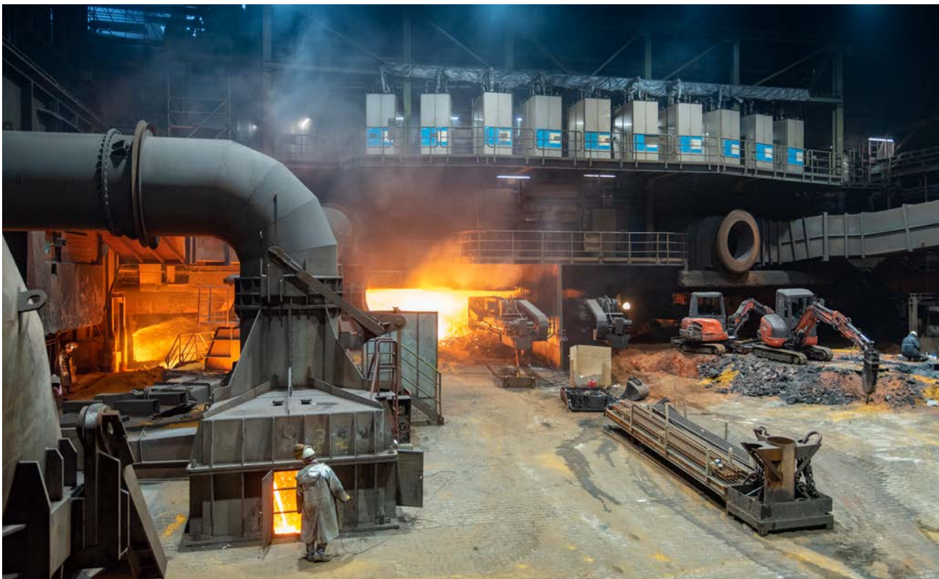
Schwelgern 1 is one of the world’s most modern blast furnaces with a potential output of 10,000 t per day. Over the course of the project, 40 SIP boxes (grey-blue in the photo) were installed on the tuyeres. The boxes inject strong intermittent impulses with technical oxygen into the coke bed in order to achieve the best possible penetration.
