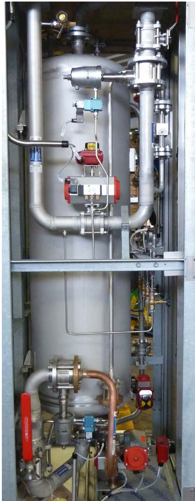
View inside an SIP box: Two type-8040 sliding gate valves were further developed over the years so that they are capable of releasing the necessary impulses with strong shock waves and have a minimum service life of one year, i.e. several million switching cycles.
