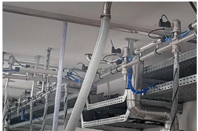
“Our pneumatic three-way valves, the so-called type 7081 3/2-way valve is perfect choice for the high cycle performance required.“ says Heiko Renn.
