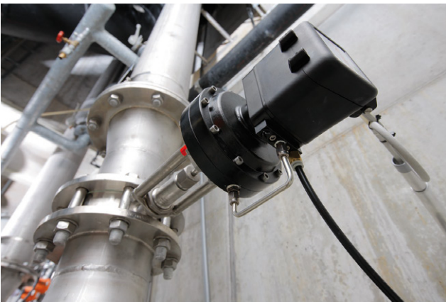
Sliding gate valve to control the oxygen content in the biological process
